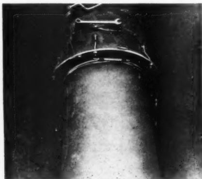
THE COMPLETED INSTALLATION Note that galvanized cable and union are insulated from pressure flange and from pipe.
